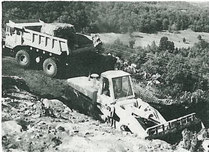
Rock and earth yield at the construction site – but unwillingly.
