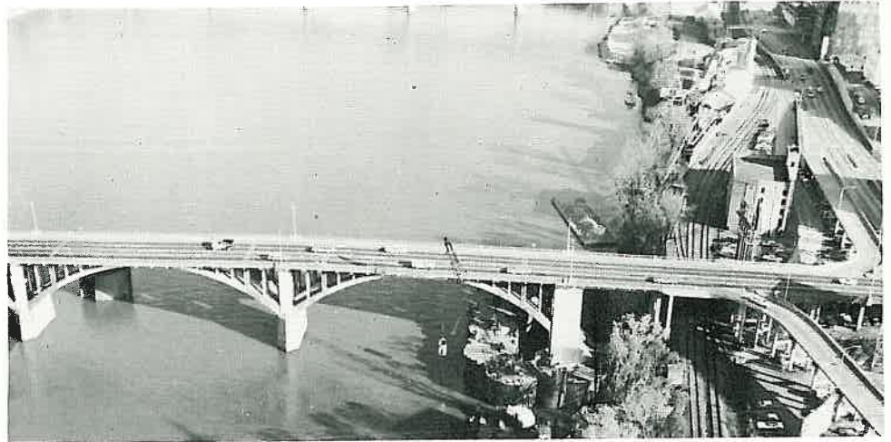
The Broadway Bridge before . . . . .
